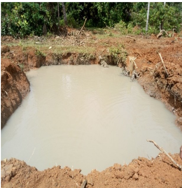
Gambar 2. Settling Pond Aktual
