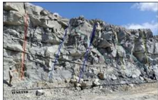
Gambar 3. Front penambangan blok B
