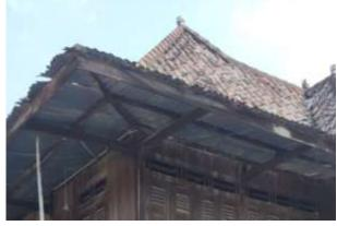
**Image 10.** The Building Frame (Top) and Roof Structure (Bottom) are Made of Wooden Joints Source: Author, 2023
