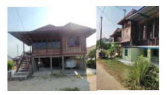
**Image 8.** Hollow Foundation Section (Left) and Foundation Section, which is Used as a Closed Room (Right)
