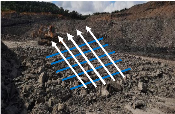
Gambar 3. Metode Cross ripping
