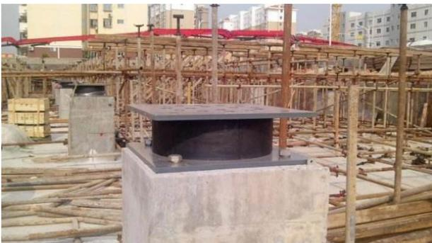
Gambar 11 Seismic Bearing (Qingdao Bless Industry And Trade).
