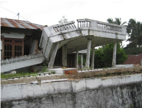
Gambar 3 Contoh Soft Storey effect .
