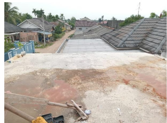
Gambar 4. Aplikasi self-compacting concrete
