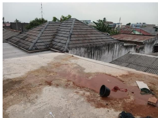
Gambar 5. Aplikasi self-compacting concrete
