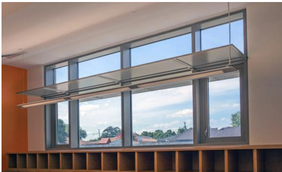
Gambar 2 Contoh Light Shelf 2 Sumber: https://www.kawneer.us/products/sun-control/inlighten-interior-light-shelf/
