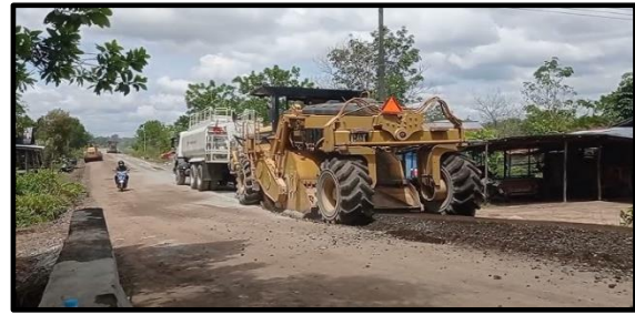
Gambar 5. Mix In Place Campuran CTRB
